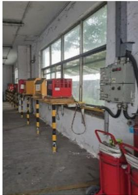
Special management of forklift charging area - independent room for isolation, configuration of fire emergency measures
