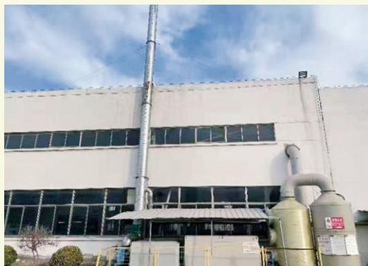
Waste gas treatment device (spray + photo oxygen + activated carbon)
