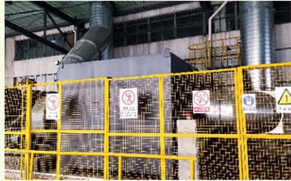
During the Reporting Period, exhaust gas emitted by the hot-melt adhesive process for box sealing at the stroller factory was collected and treated before discharge to reduce air pollution.
