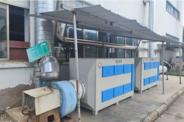
The upgraded carbon adsorption facilities
